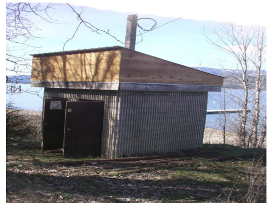
Lakeview Place Water System Pump house
