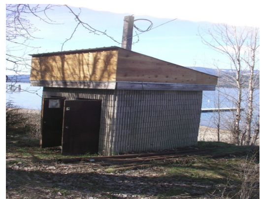
Lakeview Place Water System Pump house
